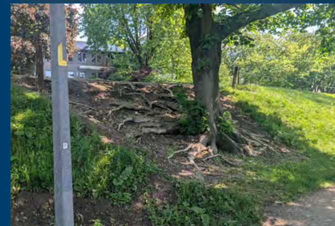
Pinch point at William Street & North Shore path
